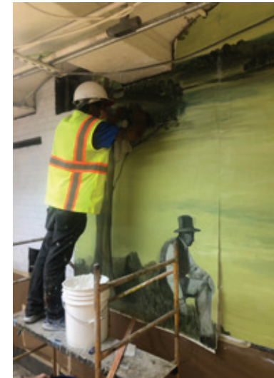
Panels being glued to brick walls.
